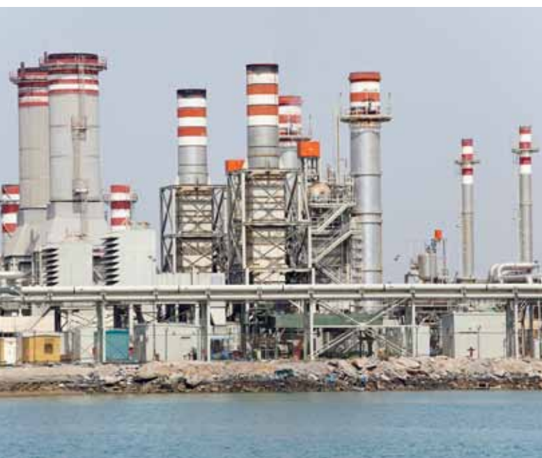
Desalination remains the most practical way of meeting rising demand for water in the countries of the Gulf Cooperation Council. © Tanuki Photography
