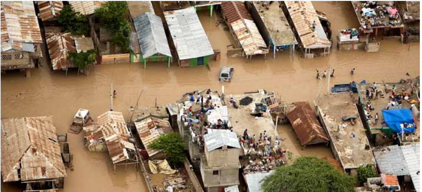
Flooded houses in the aftermath of tropical storm “Hanna”, Haiti. Better information on disaster risk is a growing priority in most regions.
